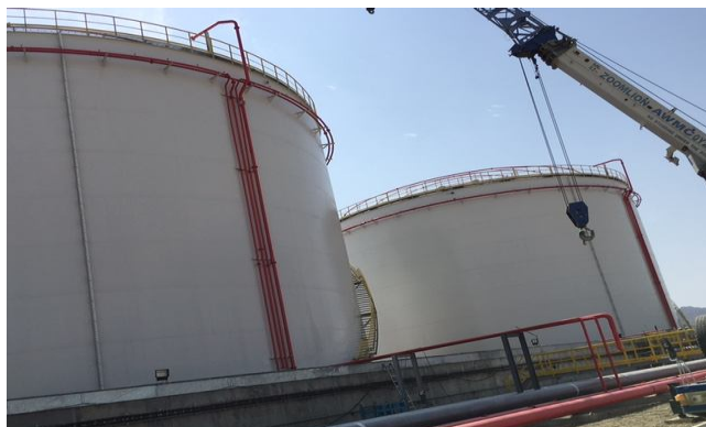
Progress of Foam Water Spray System for Oil Tanking
