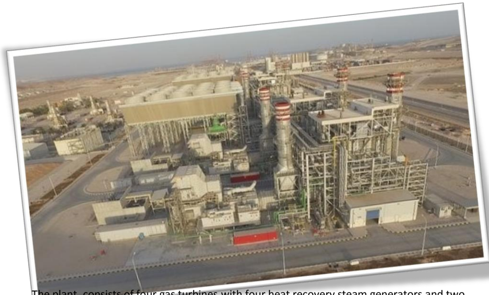
The plant, consists of four gas turbines with four heat recovery steam generators and two steam turbines.
